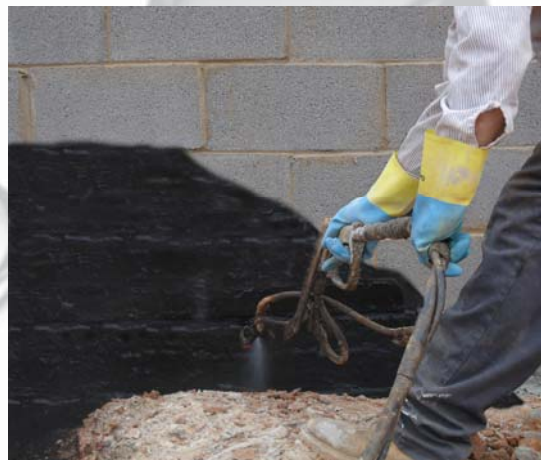
BoneDry™ XT waterproofing membrane shown with available 12" DrainMax™ foundation strip drain to make the BD1000 Waterproofing System
