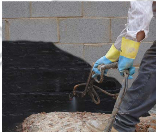
BoneDry™ WP waterproofing membrane shown with available 12" DrainMax™ foundation strip drain to make the BD1000 Waterproofing System
